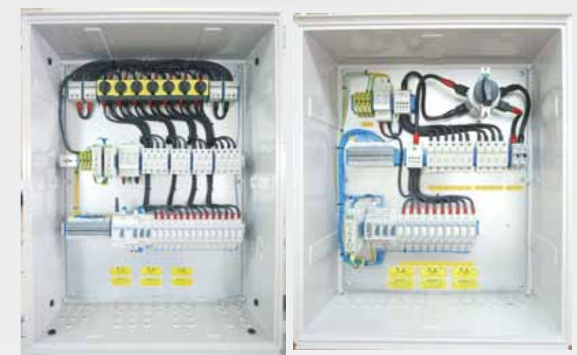
智慧型直流匯流箱 pvBos® Smart combiner box , string monitor
