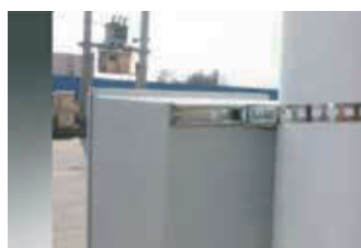
Fixed on the telegraph pole
